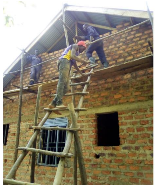
Workers completing the roof and eaves
